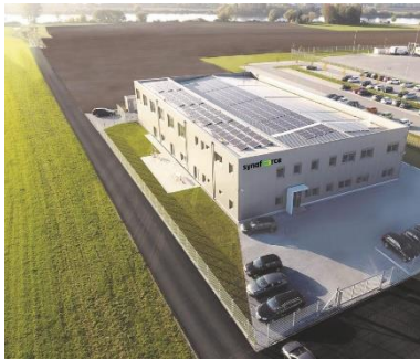
PV systems at the Hofkirchen site.
